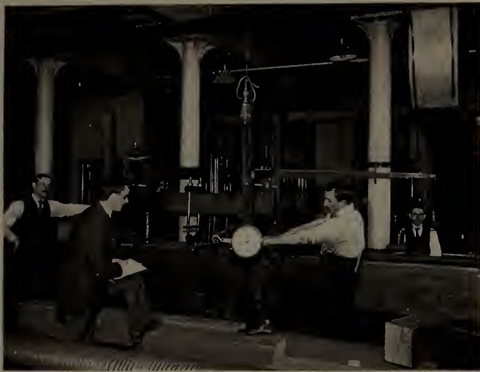
MASSACHUSETTS INSTITUTE OF TECHNOLOGY. View in the Laboratory of Applied Mechanics. Testing the efficiency of screw-jacks.
